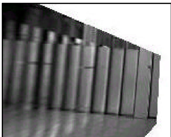
Fig. 5 Rectified image of the right wall obtained by Kanatani geometrical restoration.
